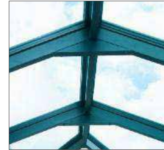
Roofs 2.5m-3.8m wide - hidden tie bar
